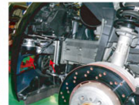
The tapping screw of air duct fixation is removed and an air duct is removed.
