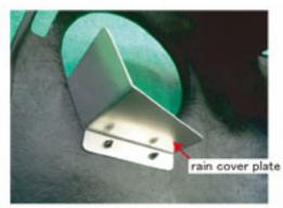
A rain cover plate is installed inside the filter case A. (Bolt C and M4 nut use)
